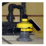
have moved toward the use of smaller storage tanks with increased automation to lower cost, and mini-bulk tanks are now a major product category. Flowline has developed a multifunction sensor to meets the needs of this growing market. The DL24 EchoPod puts non-contact level measurement, relay switch and advanced control functions in the palm of your hand.
